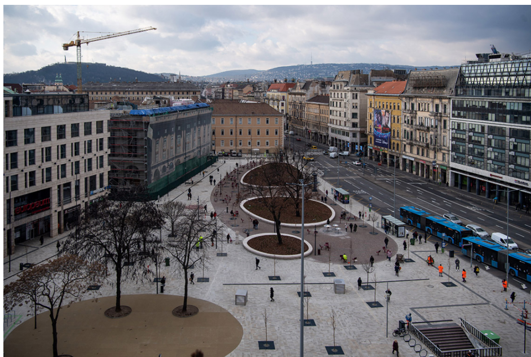
Figure 2. The renovated square in 2022. (Source: MTI/Zoltán Balogh).
